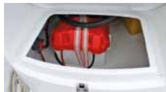
Battery locker under the forward seat
